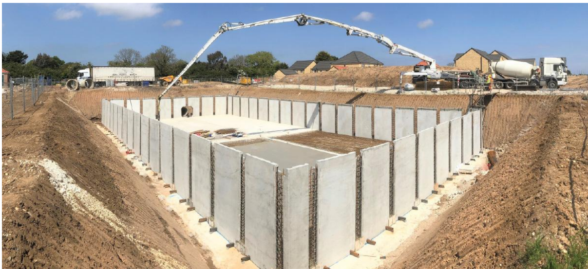
Figure 6 –Concrete Tank under construction
