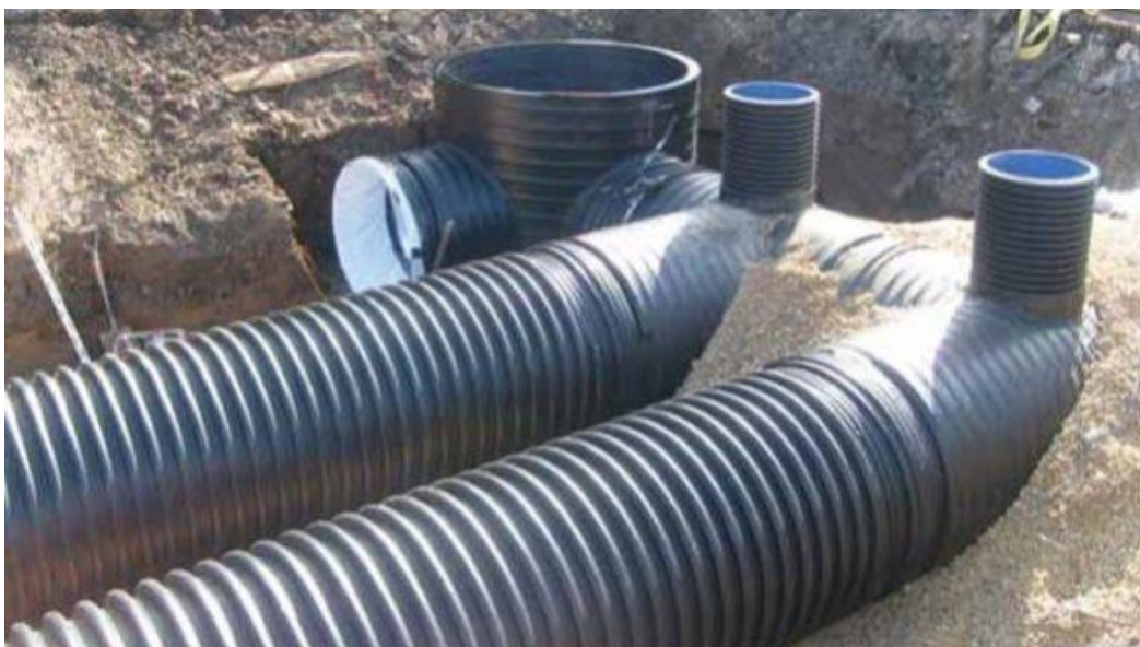
Figure 8 -Parallel Pipe System under construction
