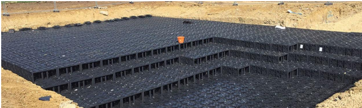
Figure 7 -Crate System Tank under construction
